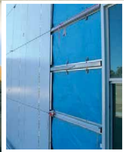
Heavy Gauge Top Hats Available in a range of sizes for fixing cladding to interior and exterior building structures.
